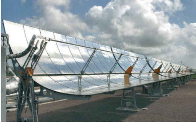
***Figure 1 – CSP Parabolic Trough Solar Collectors***
